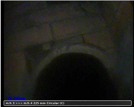
1, 00:00:04, 0.00 m Start node type, manhole, reference number: 3
