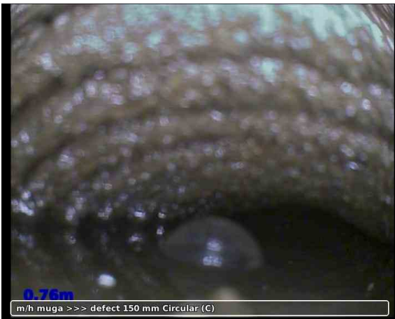
3, 00:01:24, 0.76 m Clear water level, 90% of the vertical dimension
