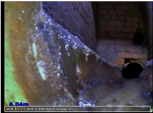
3, 00:01:02, 6.04 m Finish node type, manhole, reference number: m/h 3
