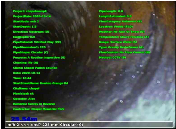
1, 00:00:03, 0.00 m Start node type, manhole, reference number: 2
