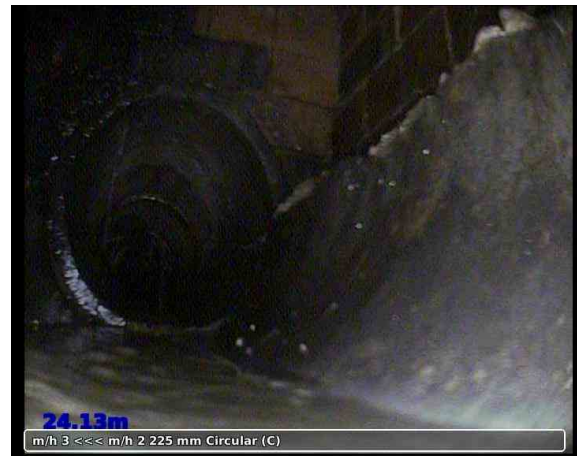
4, 00:00:19, 24.13 m Finish node type, manhole, reference number: m/h 2
