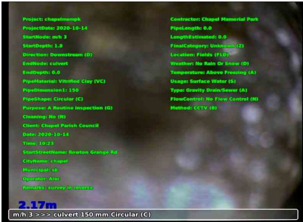
1, 00:00:04, 0.00 m Start node type, manhole, reference number: 3
