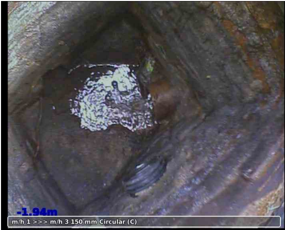
1, 00:00:04, 0.00 m Start node type, manhole, reference number: 1
